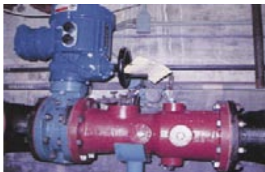
Rehabilitation Design Services
