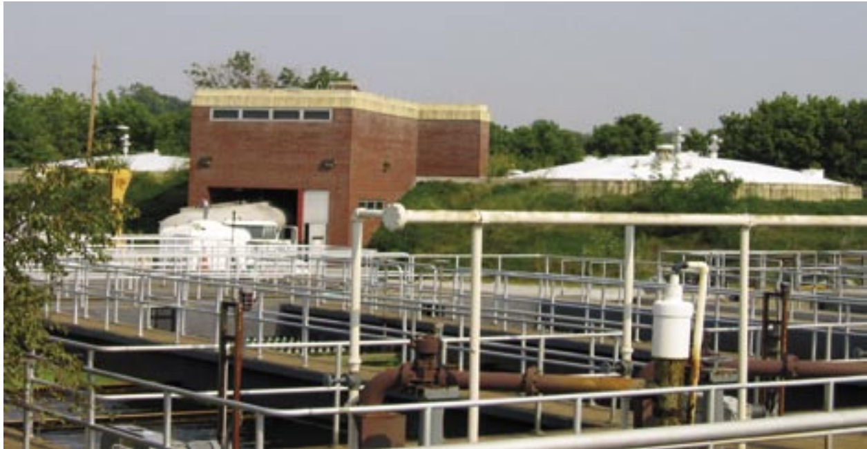
Wastewater Treatment Plant Rehabilitation
